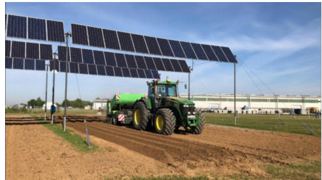
Fig. 5.24: Potatoes grown under solar panels prototype (Krinner Carport GmbH) 12
